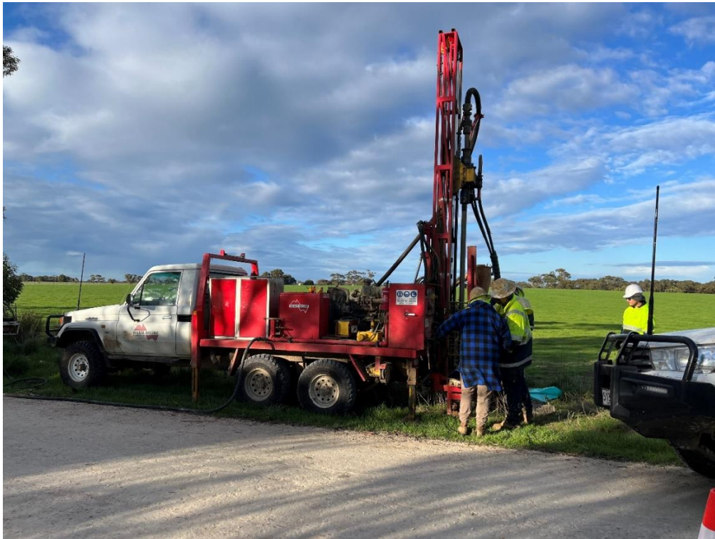
Image 1: Roadside Drilling Team on Railtz Road north of Bordertown
