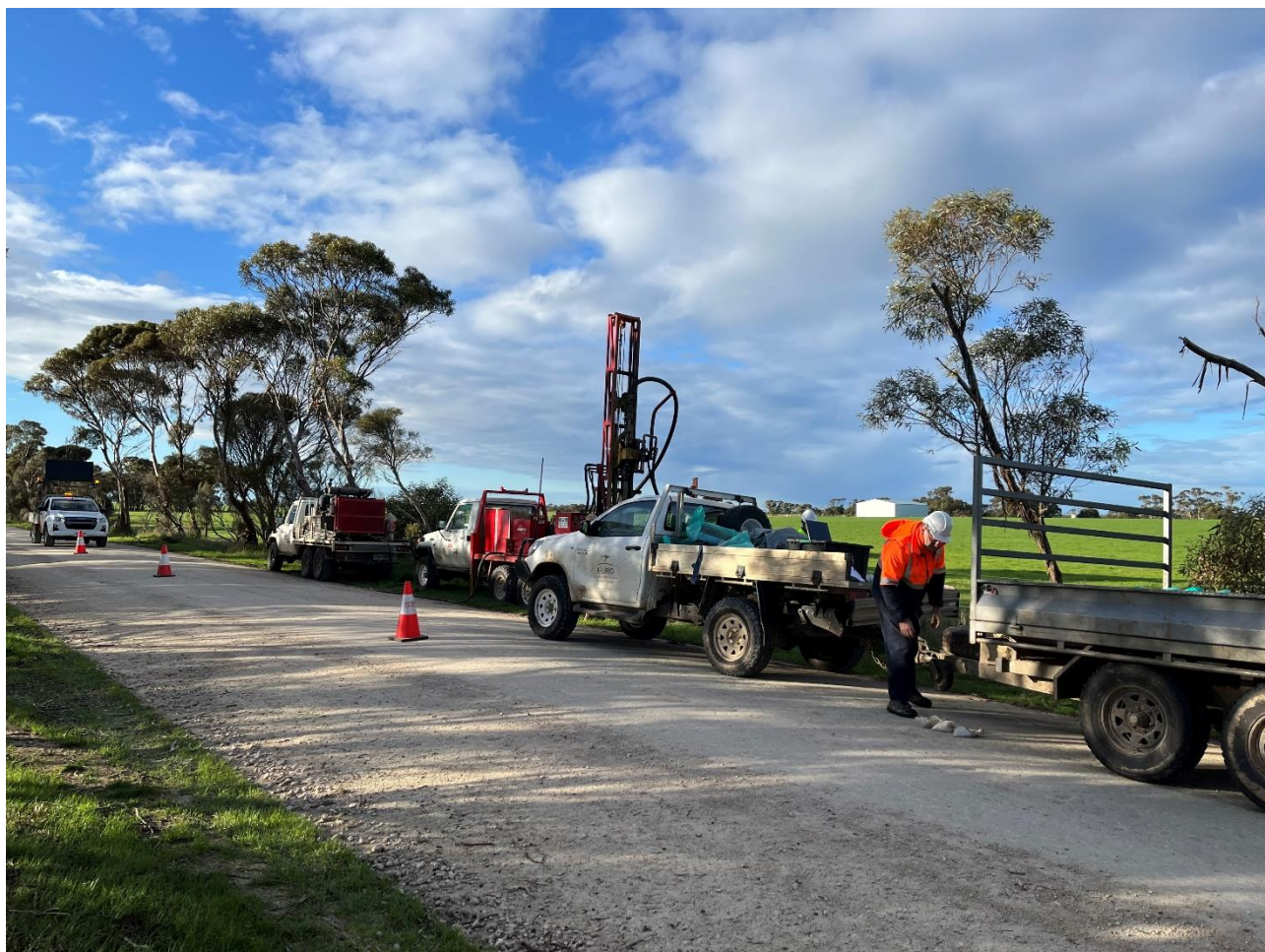
Image 2: Roadside Drilling Team on Railtz Road north of Bordertown with traffic management in place
