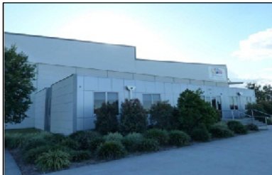
BRB's Crestmead facility
