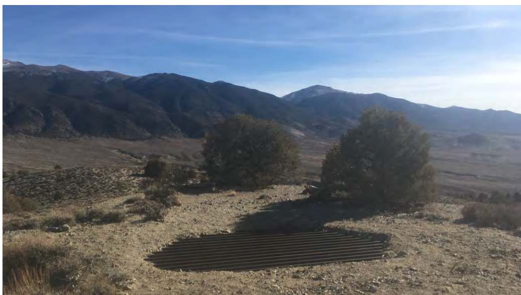
Figure 29 - A steel grate placed over a shaft of unknown depth at Caisson Project.
