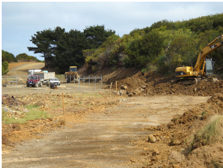
Mine site preparation of land acquired on King Island.
