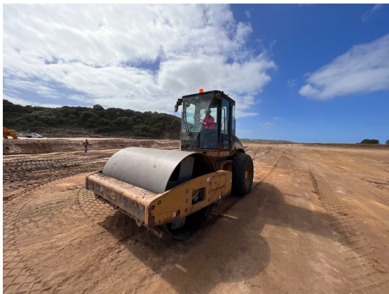
Compaction rolling of process plant area: Mar 22
