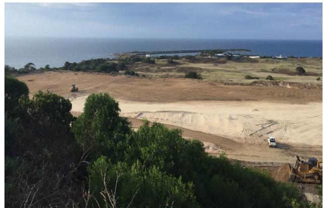
Process plant earthworks nearing completion: March 22
