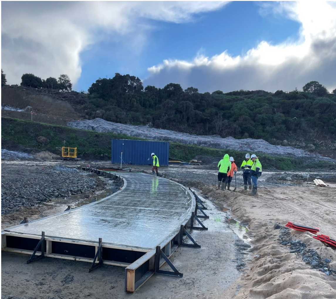
Figure 1. Concrete Installation Works for Fine Ore Bin Slewing Conveyor
