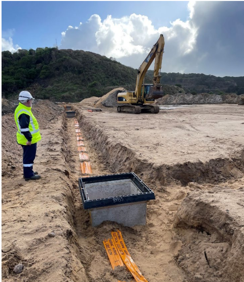
Figure 4. Process Plant Electrical Conduit Installation
