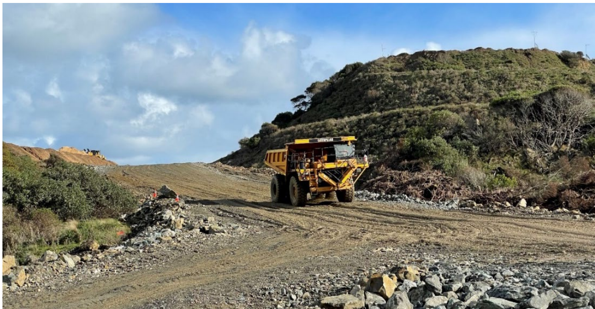
Figure 2. ROM Haul Road Alignment and Leveling Works
