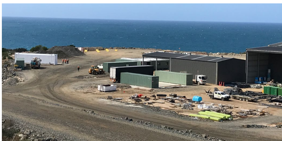
Figure 6 - Construction of warehouse, fixed plant workshop, fuel storage and go-bay area.
