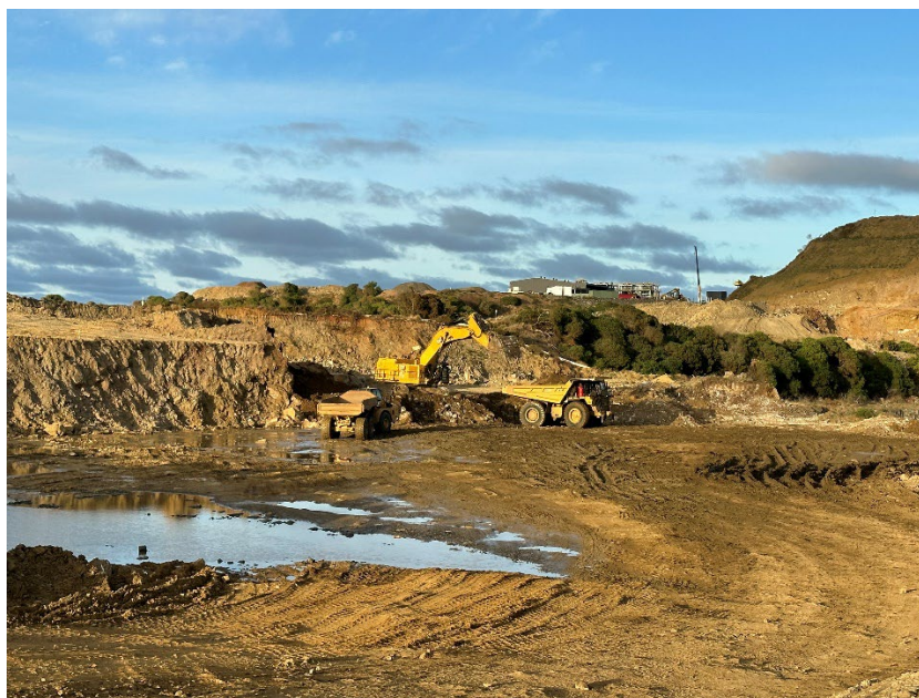
Figure 5 - Pre-stripping activities on the eastern side of Dolphin Pit.
