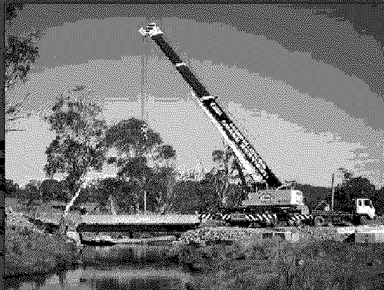
Lifting bridge sections into place at the Ruby Mine
