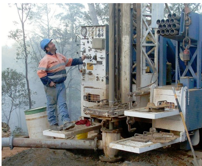
Ten inch Percussion Drilling in Progress
