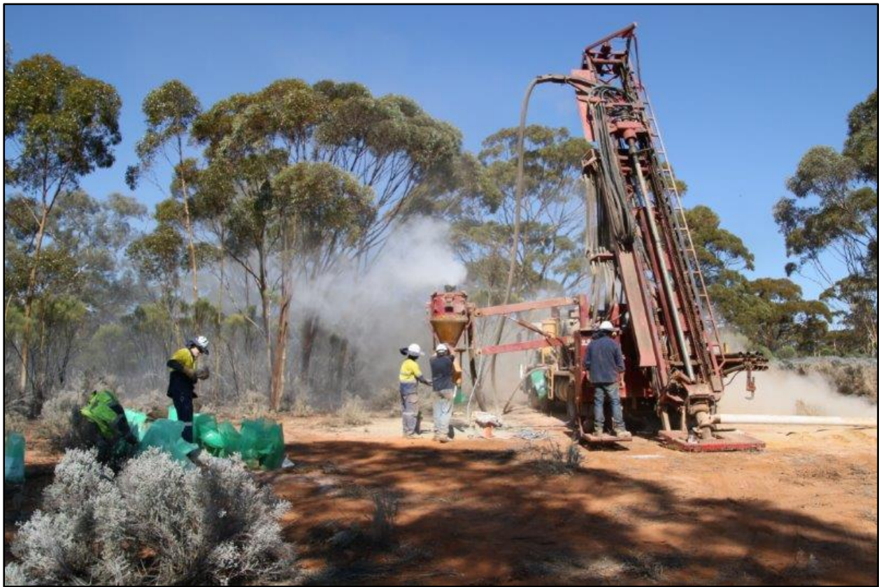
Figure 2: RC Drill Rig at the Zuleika JV.
