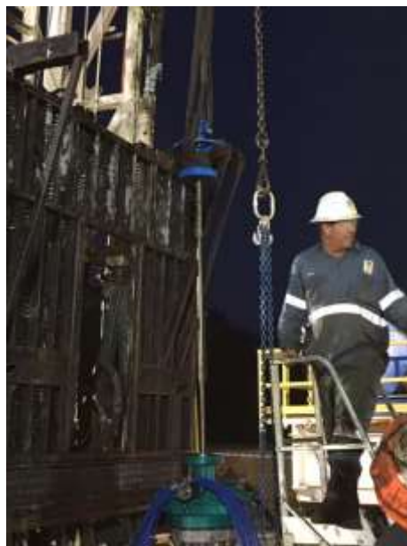
TDC Rig 4 at Nyanda-4 27.11.2020
