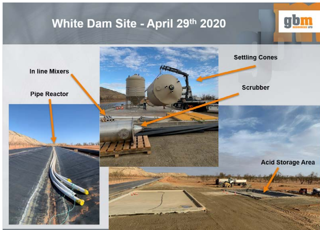
Figures: White Dam Heap Leach Gold Project – New SART Plant Site
