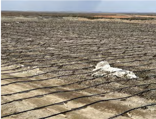
Figure 11: Irrigation on Phases 1,2 & 3 completed and now under cyanide irrigation.
