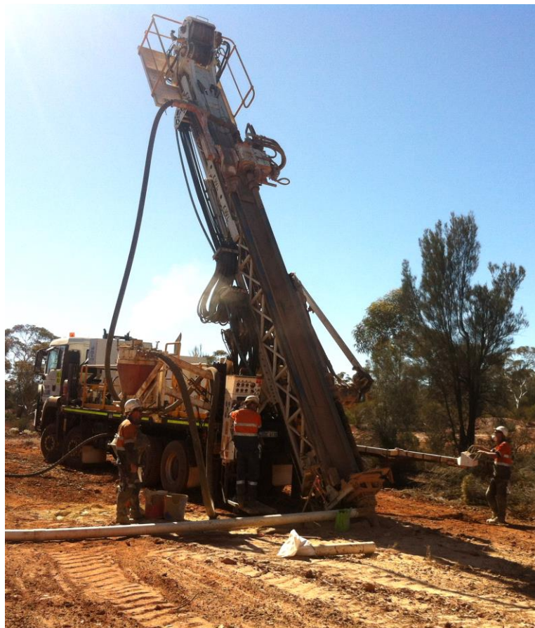
RC Drill Rig at Balagundi
