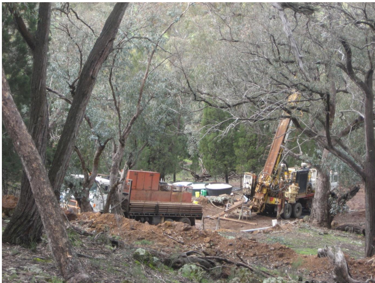
Figure 1. Core Drilling at Copper Hill
