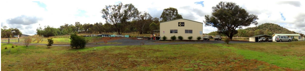
“Coppervale”, with Buckley’s Hill and Copper Hill in the background. GCR’s core shed and office facility at Copper Hill near Molong, NSW.
