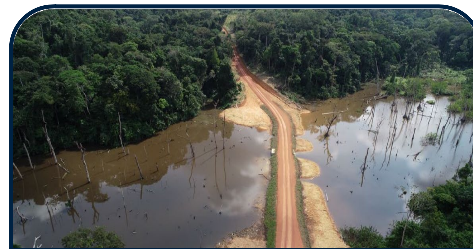
Resurfaced Tsengué Base Camp access road.
