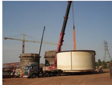
ERECTION OF TANKS AT WERGO
