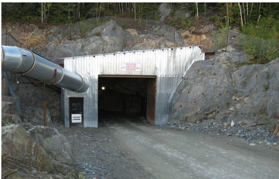
Figure 2 - Rocmec underground mine portal access (current)
