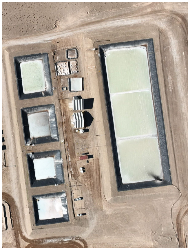
Figure 4: Aerial view of existing pilot plant
