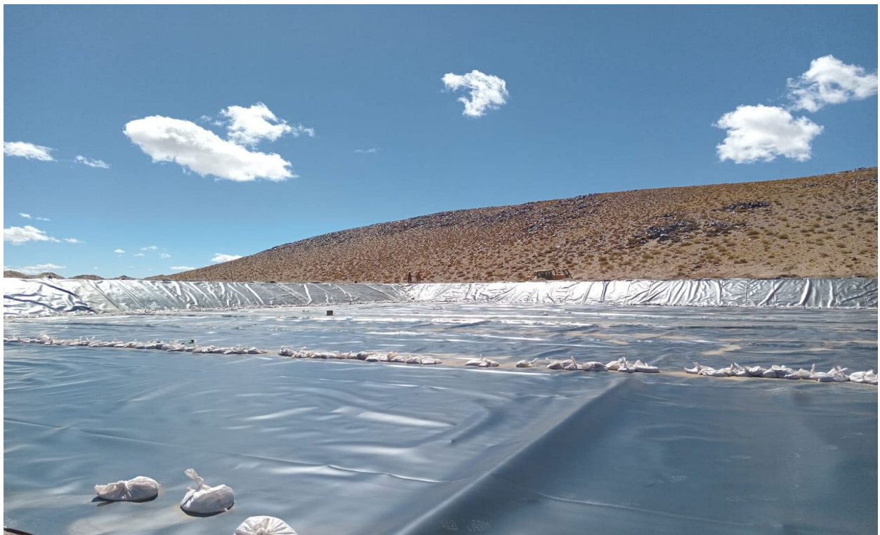
Liner installation commencement
