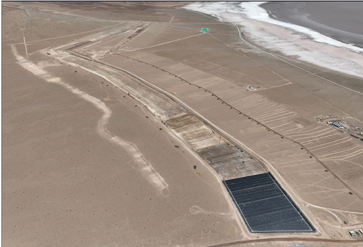
Overall progression of liner installation on Pond 1
