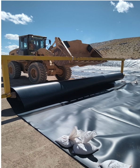
Liner installation process
