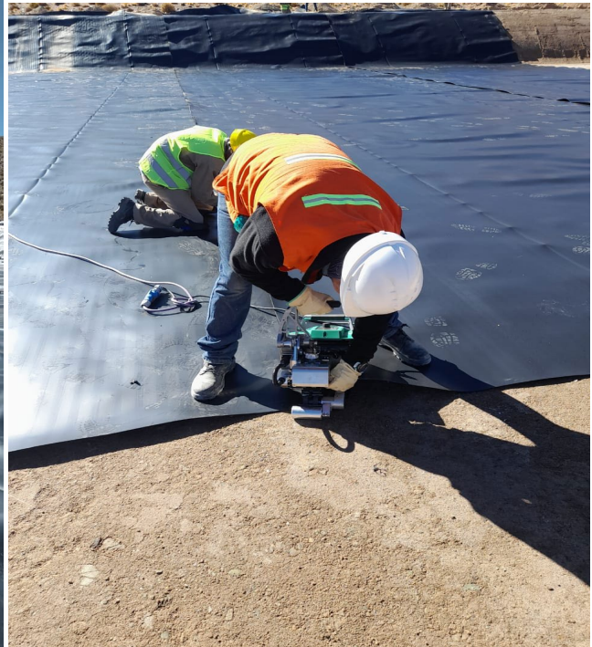
Liner installation process
