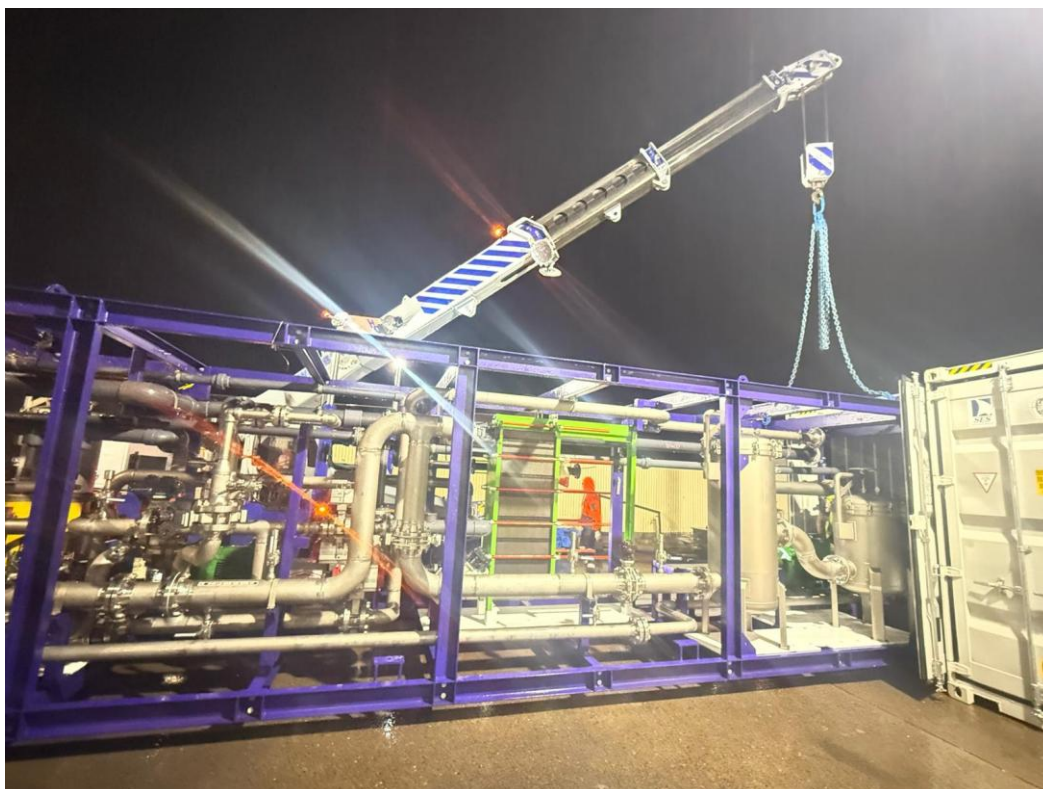
Figure 2. Load out of nano-filtration plant
