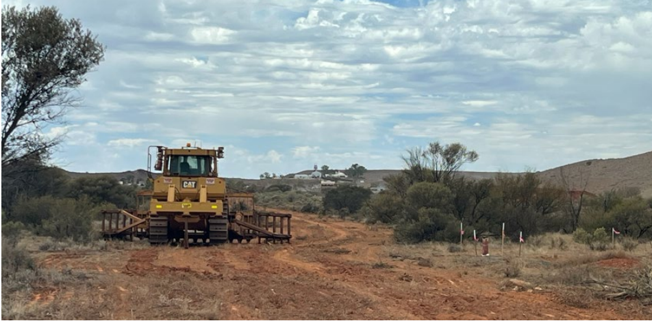
Figure 6. Tower Hill - Clearing of services corridor underway
