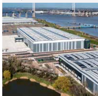
Crossways Commercial Park, Greater London, UK.
