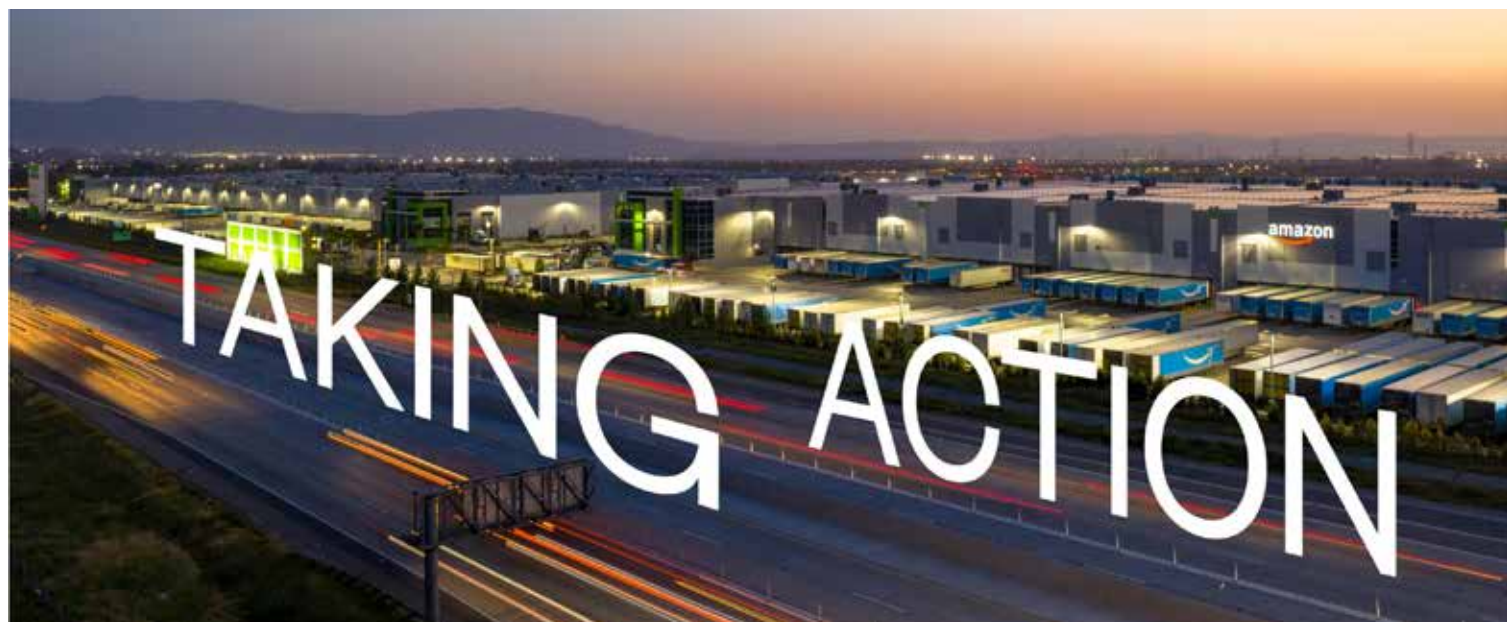
Goodman Commerce Center Eastvale, Los Angeles, USA.
