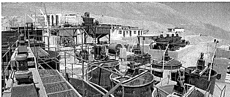
The Mollehuaca Gold Plant Peru-October 2013: Production soon.
