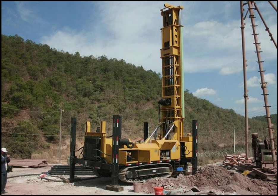
Figure 1: An Atlas Copco CS14 Drill Rig
