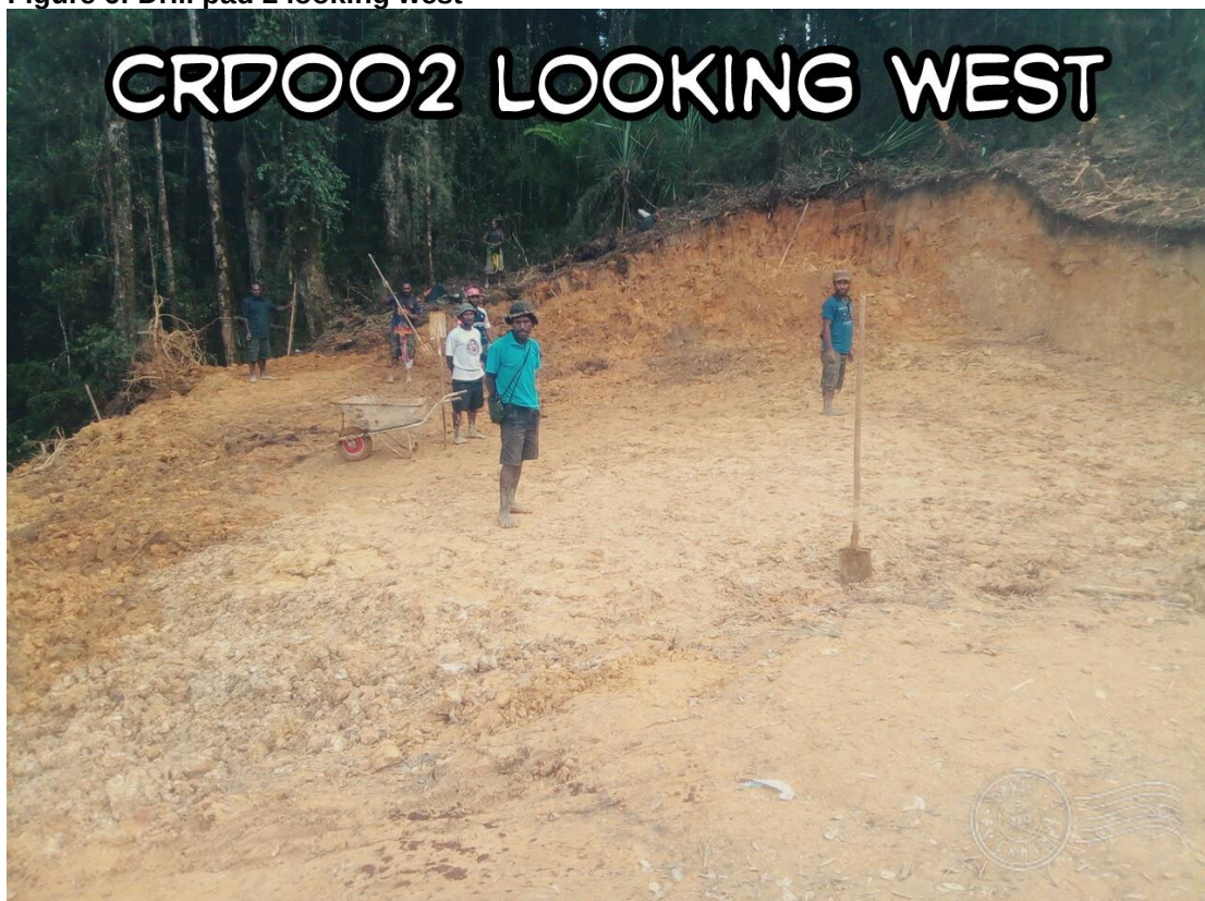
Figure 6: Drill pad 2 looking west
