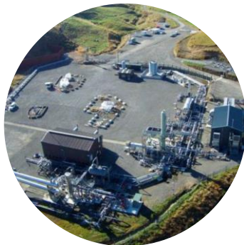
Creating fuel and plant flexibility
