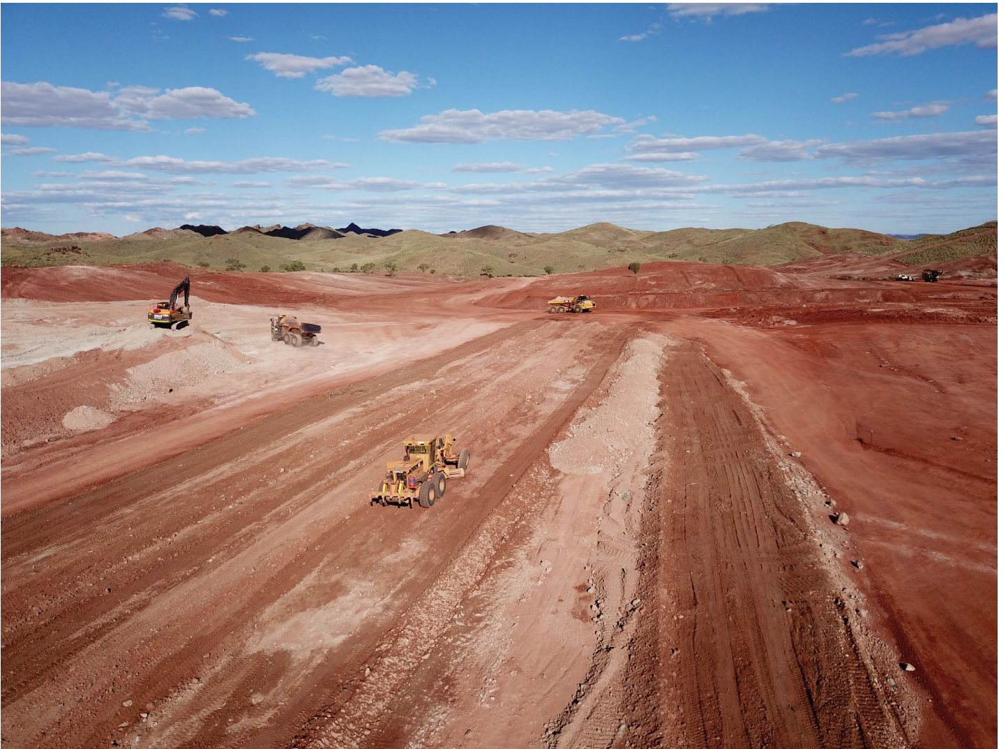
Figure 2: Bulk earthworks at process plant well underway
