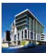
SJM Building, SW1: 32 Cordelia Street, South Brisbane
