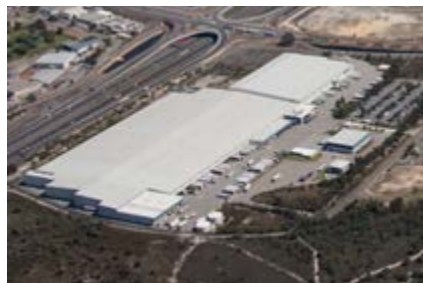
20 Colquhoun Road, Perth Airport, Western Australia
