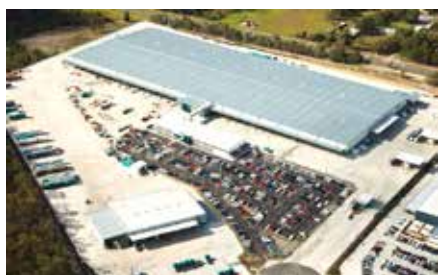
Toll NQX, Karawatha, QLD
