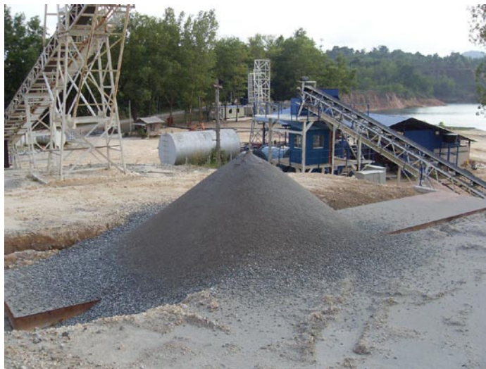
Figure 1: Bukit Ibam processing plant site and crushed ore
