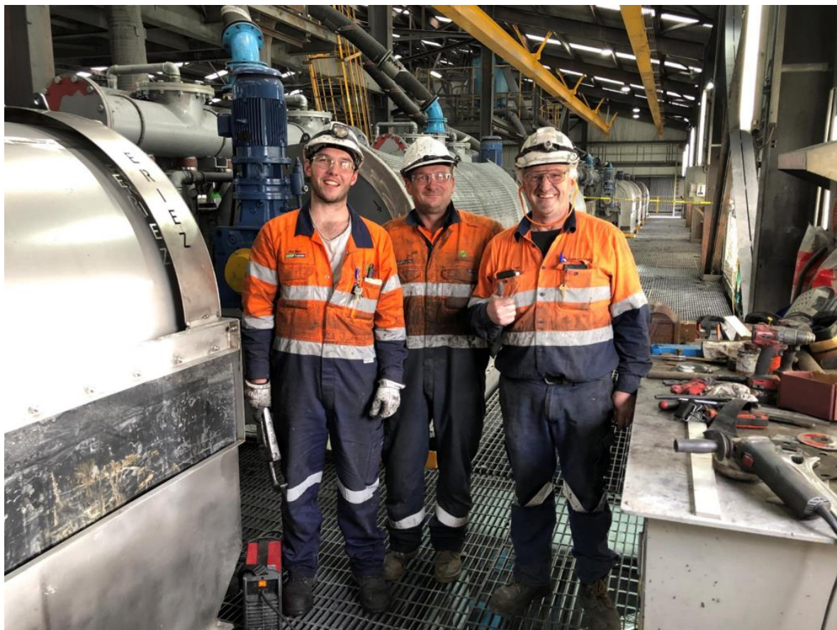
Completion of Rougher Magnetic Separator installation
