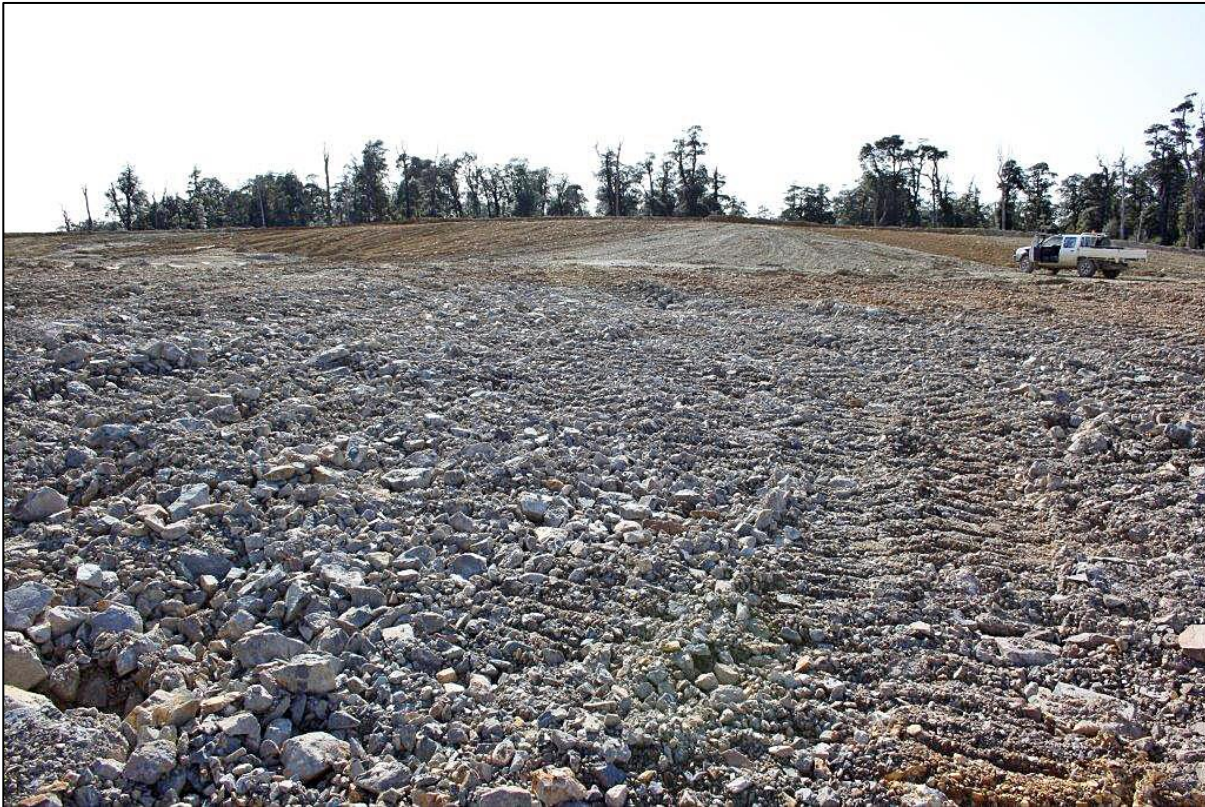
Figure 1: Rehabilitation works underway at the Que River Mine site
