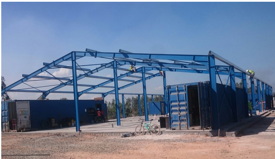
Figure 2: The Graphmada workshop preparing for roof installation.
