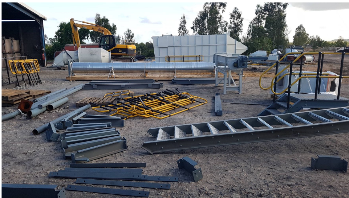
Figure 3: MDS installation underway.
