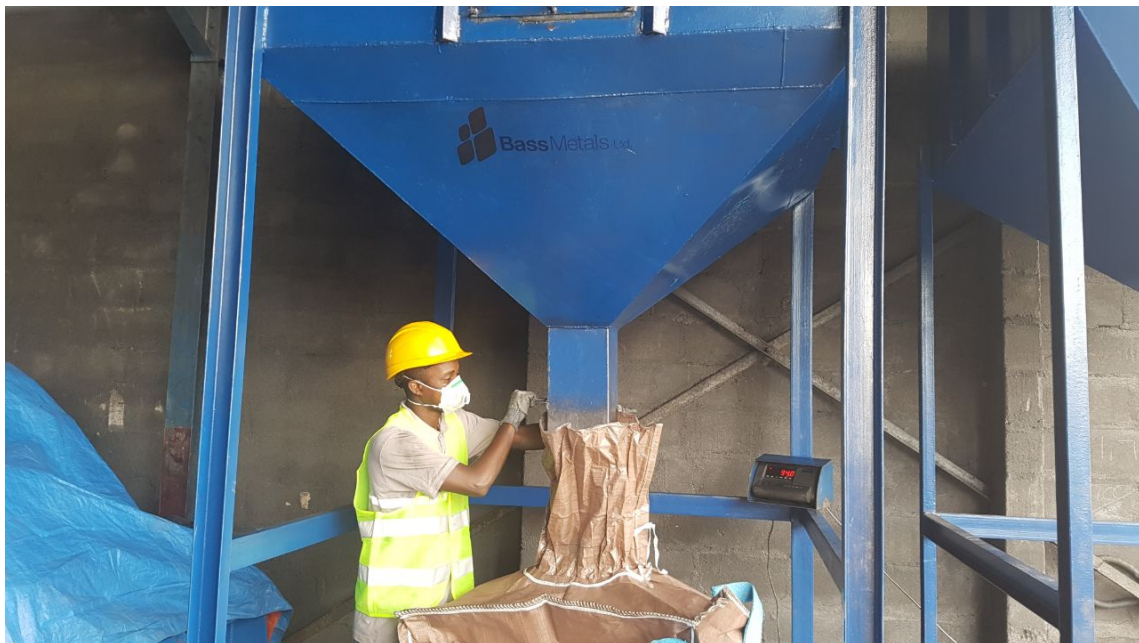
First production from the recommissioning process.
