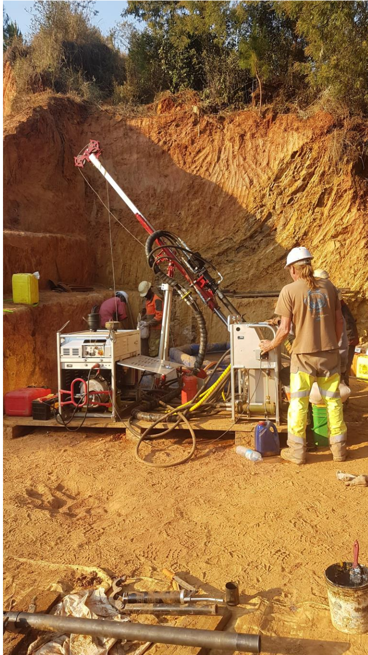
Figure 1: Drilling at Millie's West.
