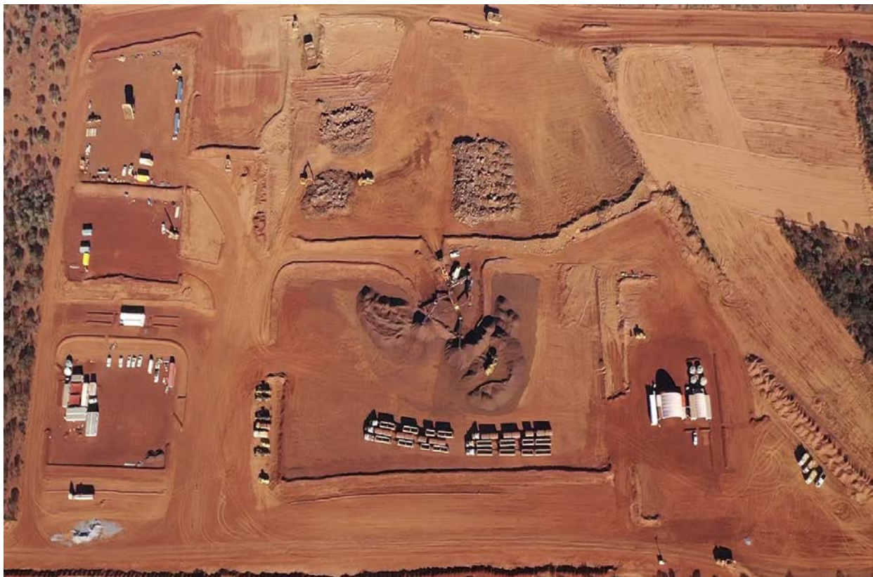
Figure 2: C4 Mine Site works with Trucks lined up ready to be loaded.
