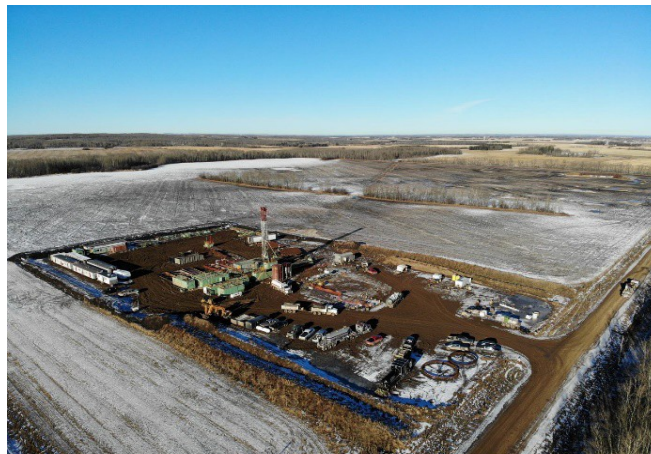
Figure 3 - Rex-3 during drilling
