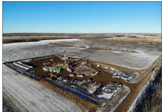
Figure 3 - Rex-3 during drilling
