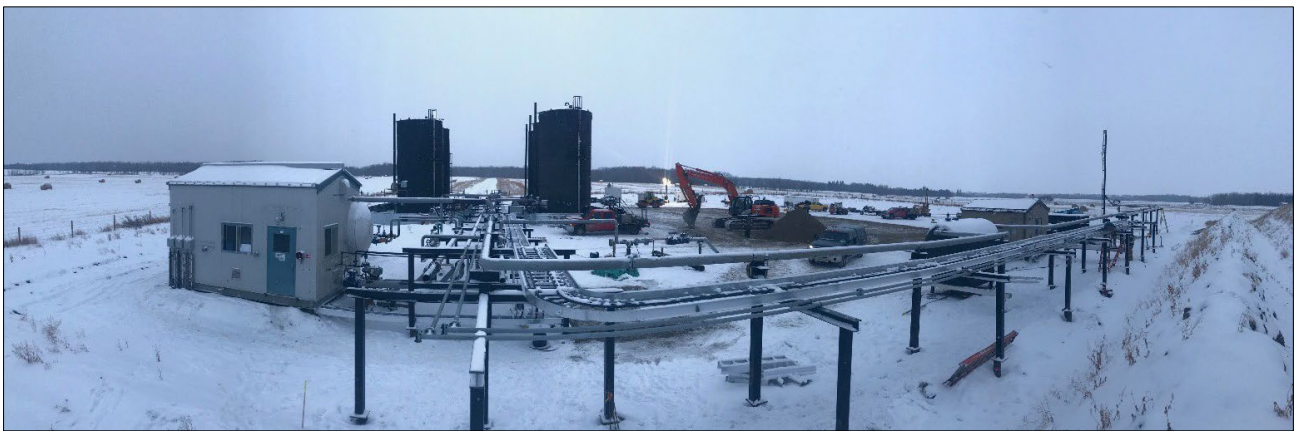
Figure 5 - Installed and commissioned upgraded Wizard Lake Facilities
