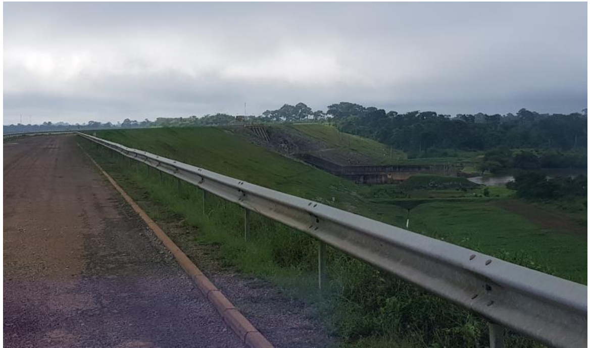
Figure 5.3_1 Hydro-Electric Dam at Buyo (Source: Sahara 2021)
