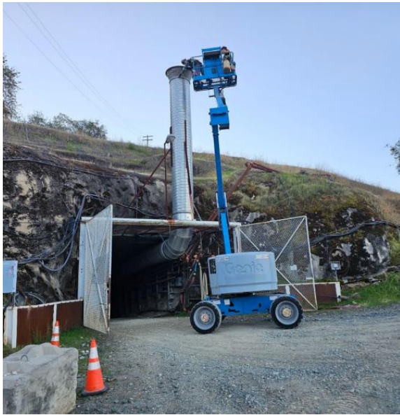
Figure 8: 4x4 articulated boom, checking ventilation tower 8 .
