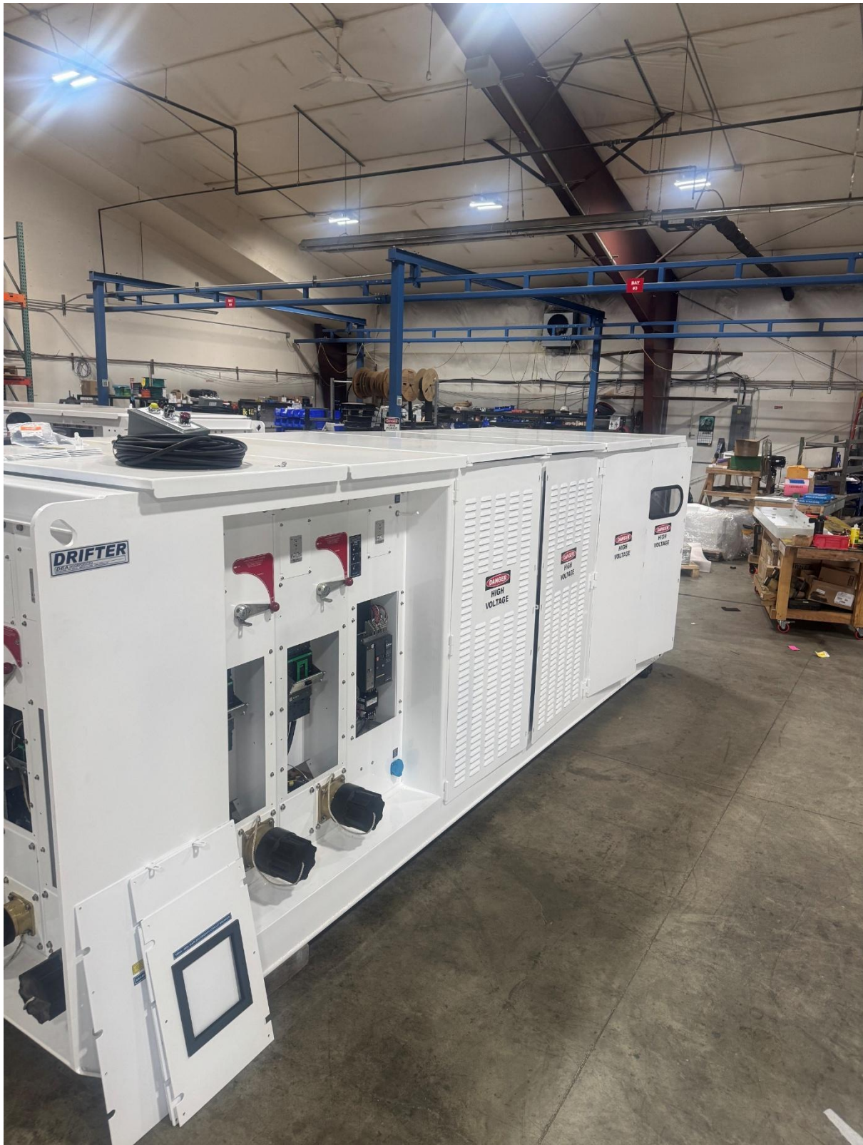
Figure 2: Haranga MPC under construction by supplier (to be placed underground at XC7).
