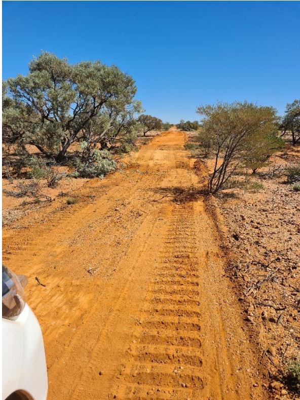
Figure 3: Access track construction
