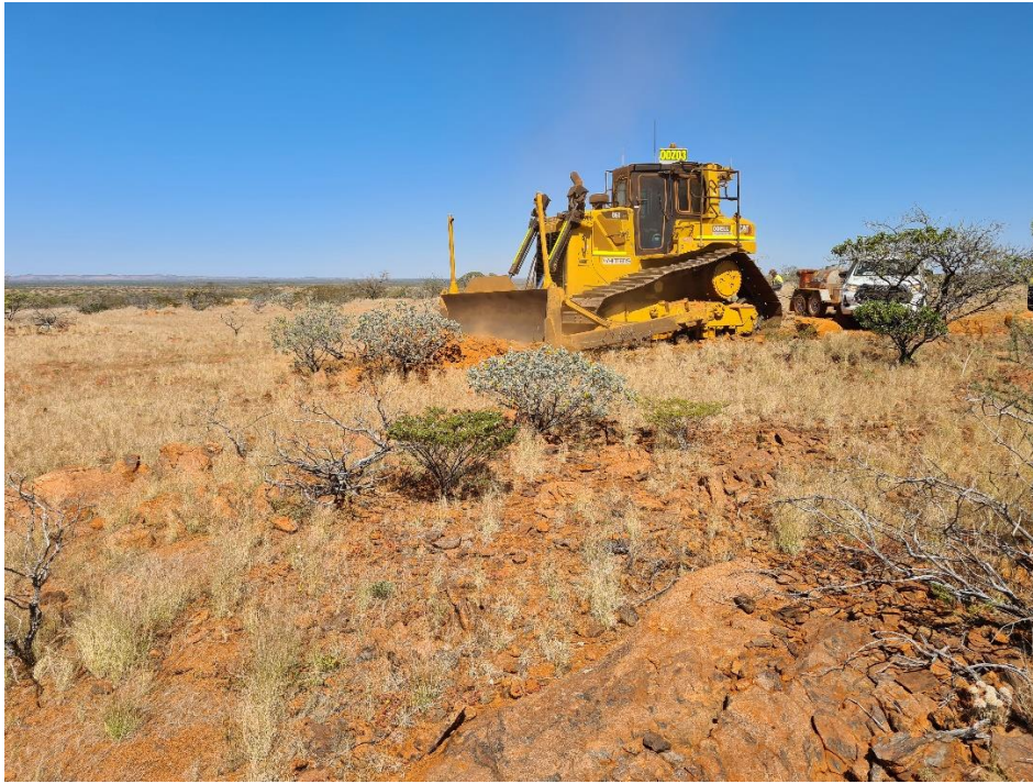
Figure 7: Dozer commencing early works
