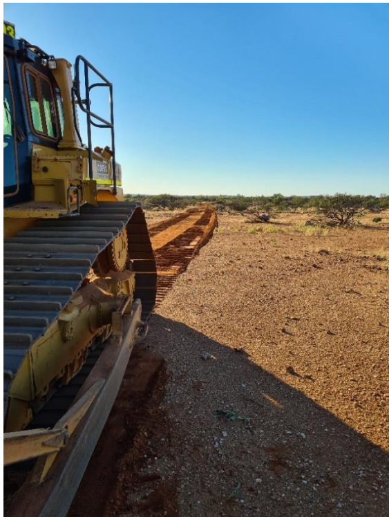
Figure 5: Site access track clearing
