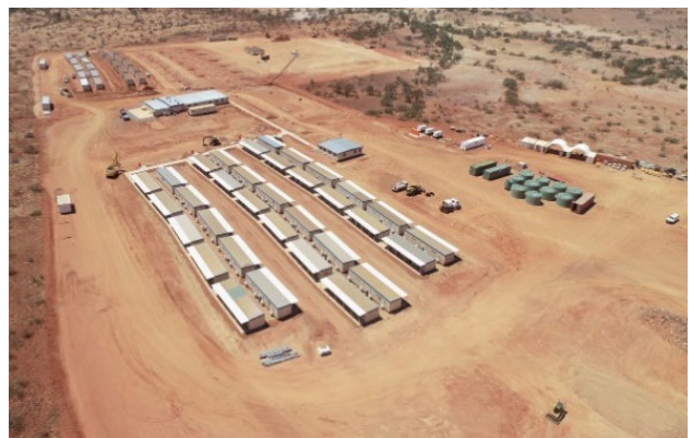
Figure 3. Kurrbili Accommodation Village: Phase 1 and 2 taking shape.
