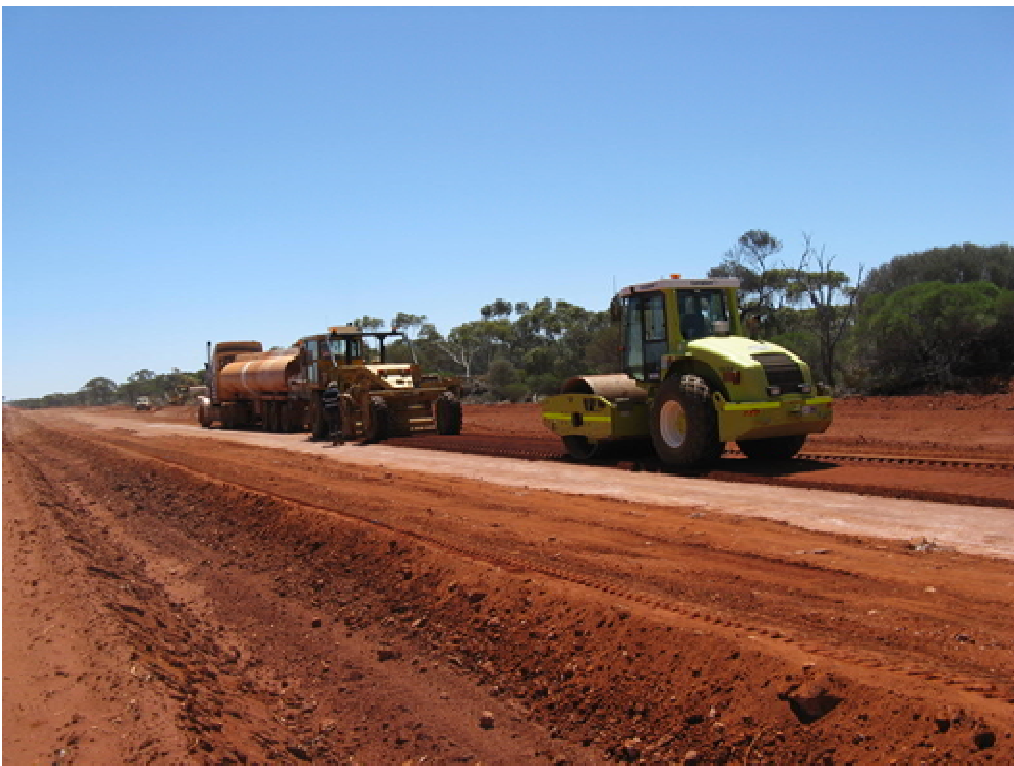
Figure 2 & 3. Anglo Saxon Haul Road construction – September - October 2017
