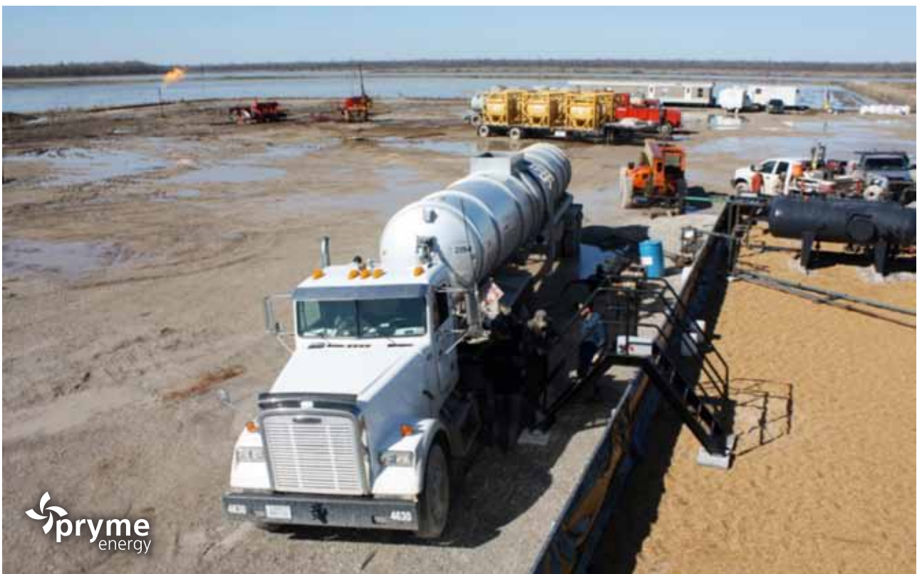
Oil being sold and gas being flared from the Deshotels 20-H No.1 well in Turner Bayou
