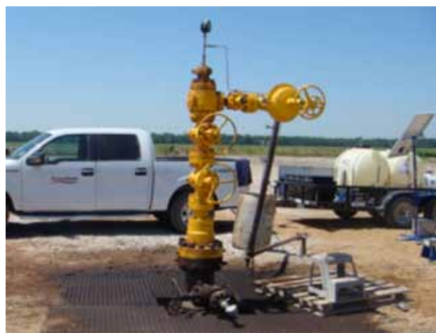
Deshotels 20H No. 1 Production Well Head
