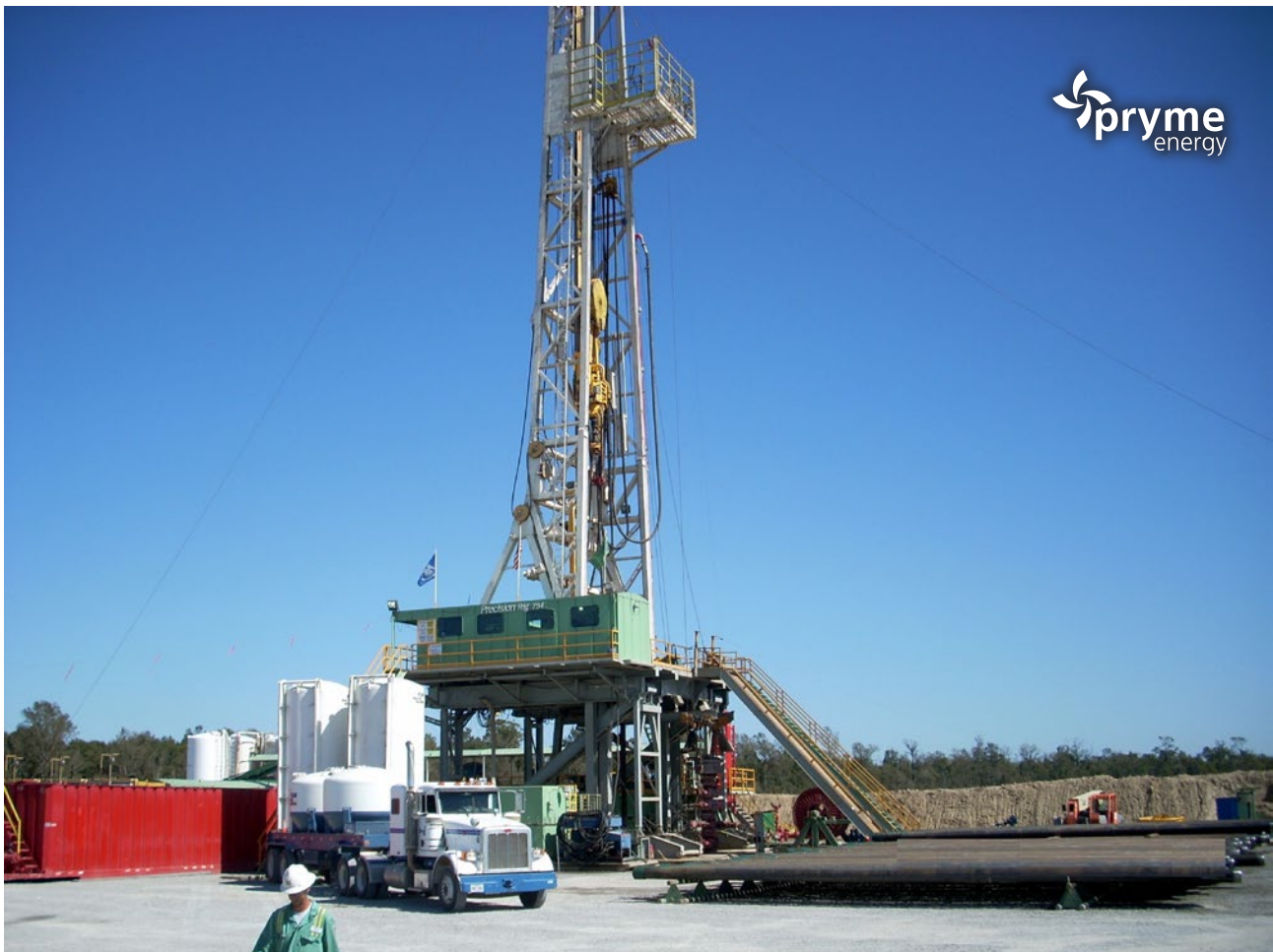
Drilling the Rosewood Plantation 21H well
