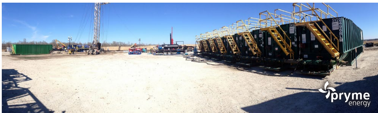
Work over rig running tubing and flow back tanks on Rosewood Plantation 21H well site
